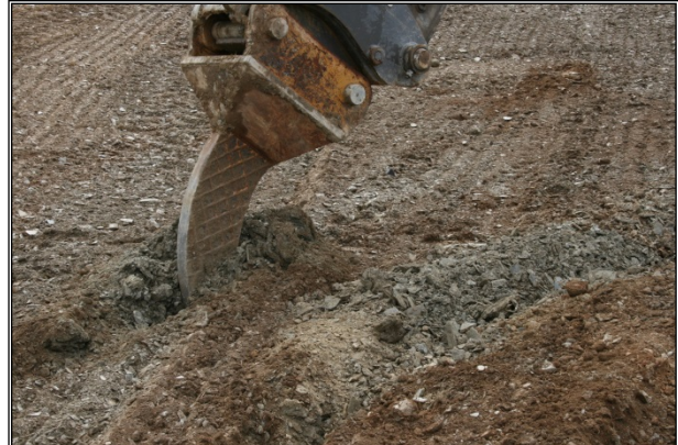
Inset 4 Tracked excavator with single rigid tine (Left) and Single rigid tine in use (Right)
